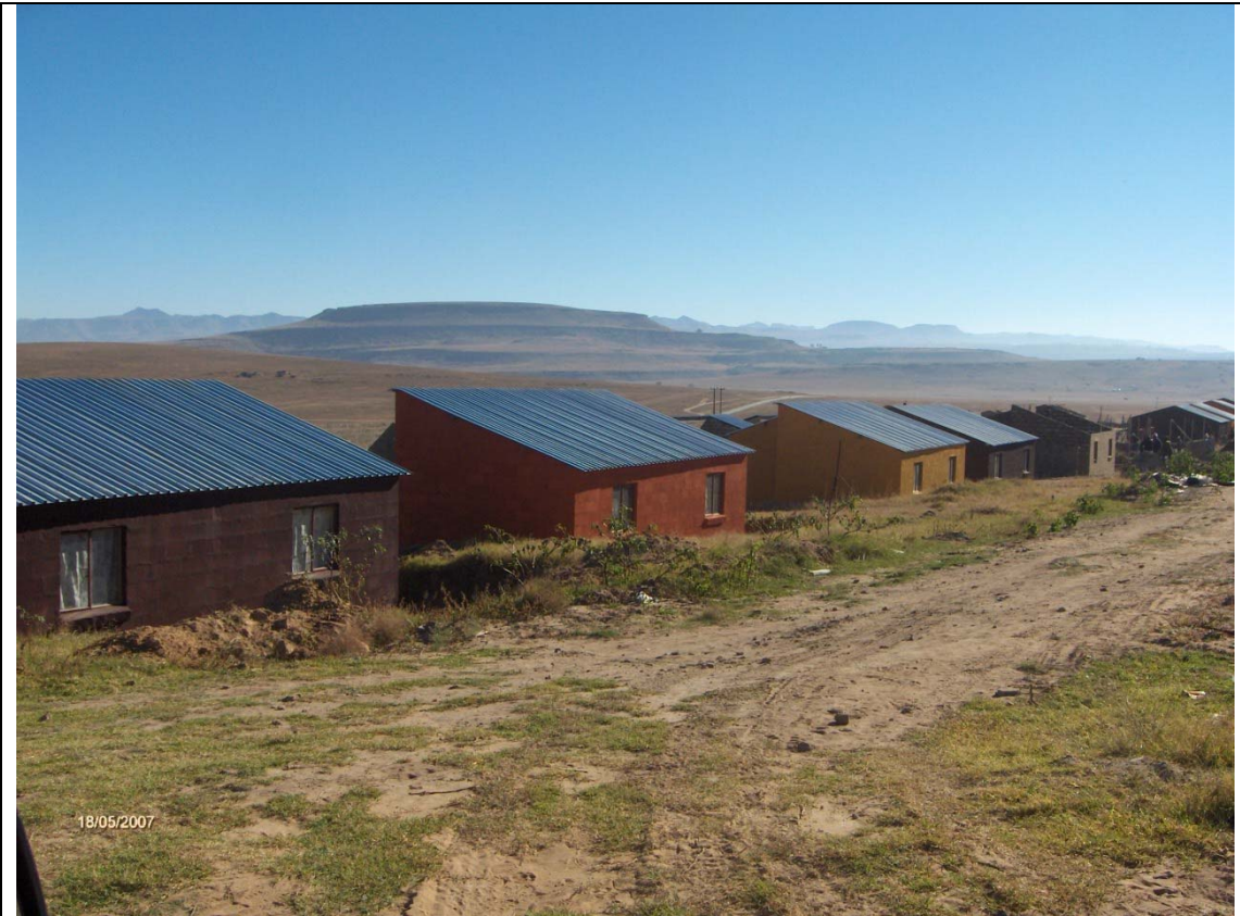
Pic2: Deep cut on which houses are built
