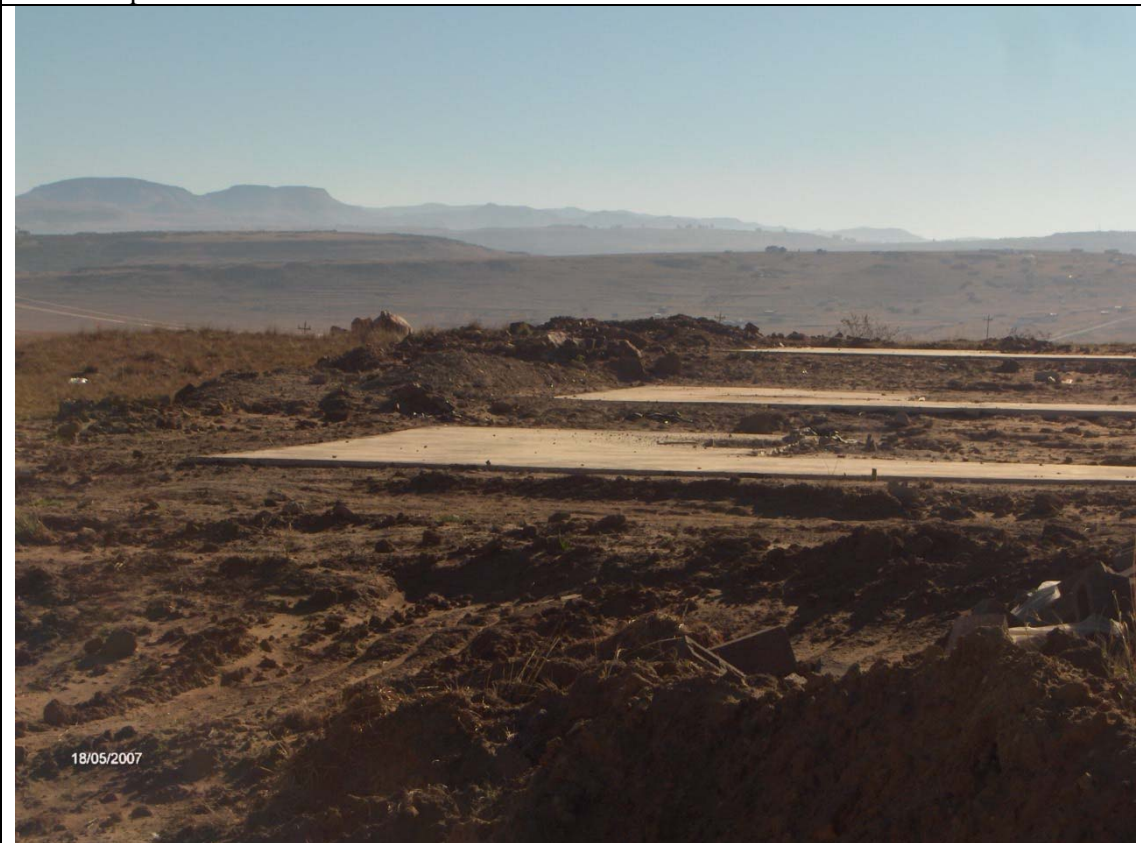
Pic3: Surface beds cast on cut
