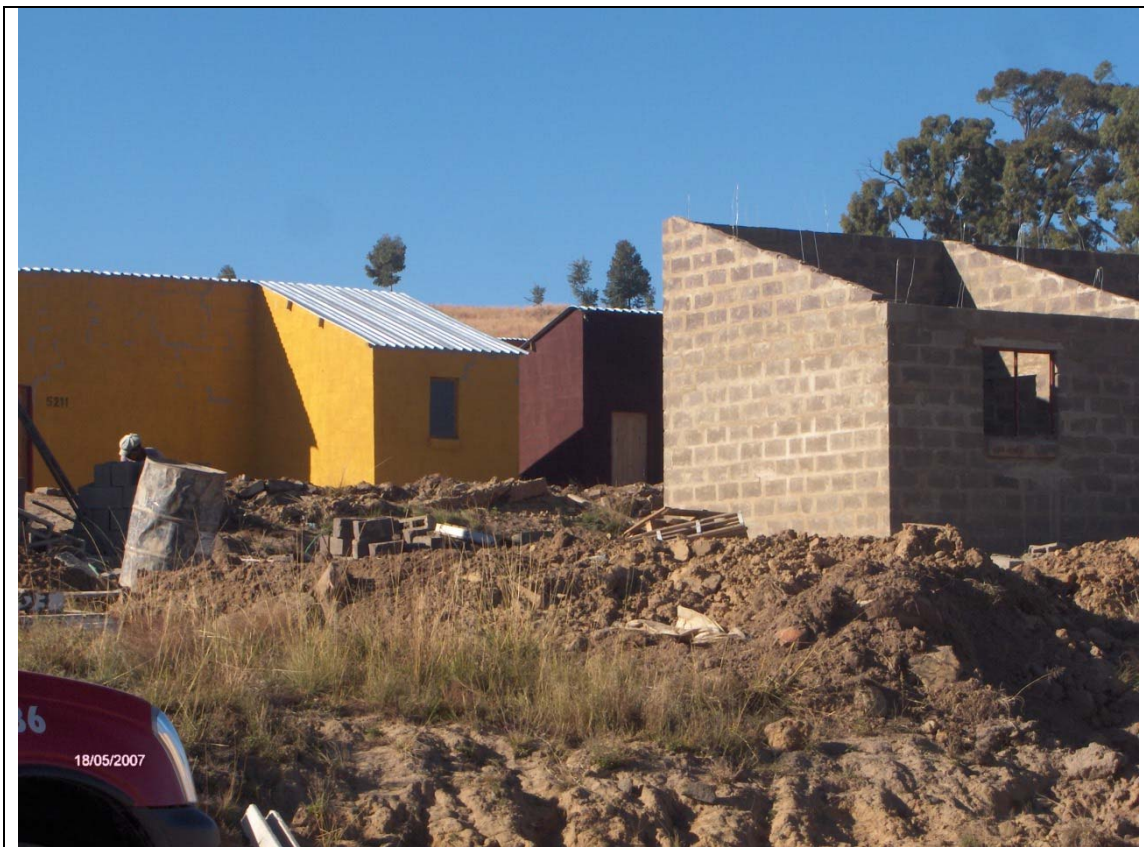
Pic1: Steep slope of the terrain
